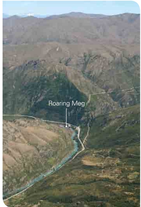
Approaching the Roaring Meg power station inbound along the Kawarau Gorge from Cromwell.
